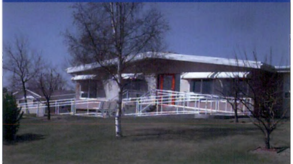
Bashway Valley Lodge (after renovation)
