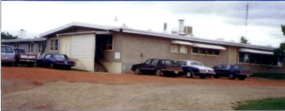
North-West corner (before renovation)
