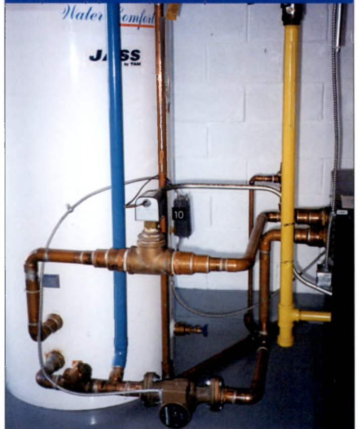
New hot water storage tank and boiler (right). Note the circulating pump in bottom pipe, flow switch in top pipe.
