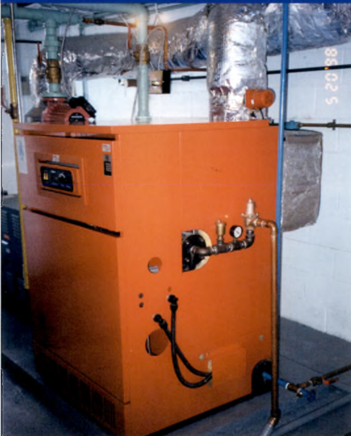
New space heating boiler. Note the motorized insulated flue damper.
