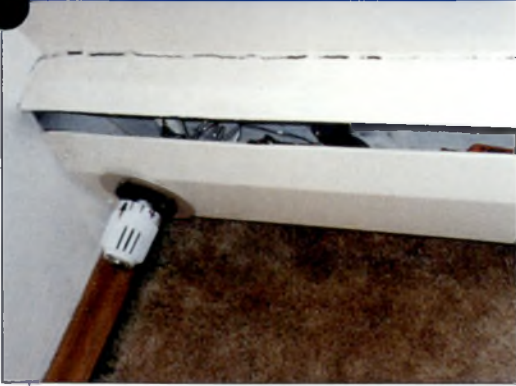
Typical baseboard heater with thermostatic radiator valve
