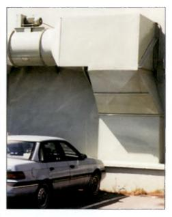
*Compliance with B.C. Building Code:* The ducts from the old east fan system go through the top level of the parkade. By installing an exhaust louver at the old duct and
