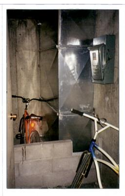
10 per cent of the lower explosion level (LEL) concentration, the fans turn on after two minutes. An alarm goes off if propane reaches 20 per cent LEL.
